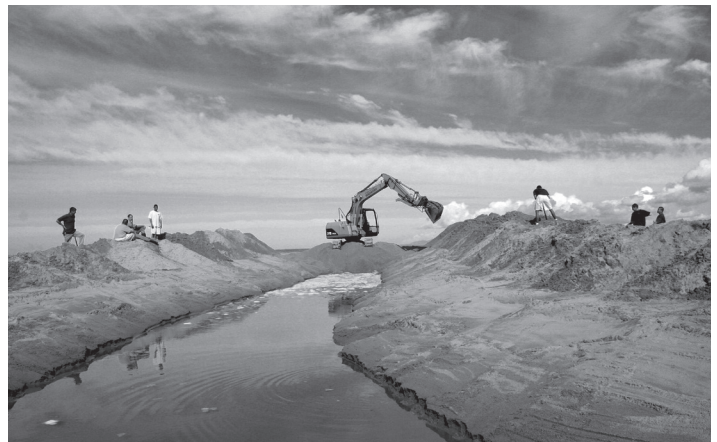
The second attempt: an excavator clears the channel
