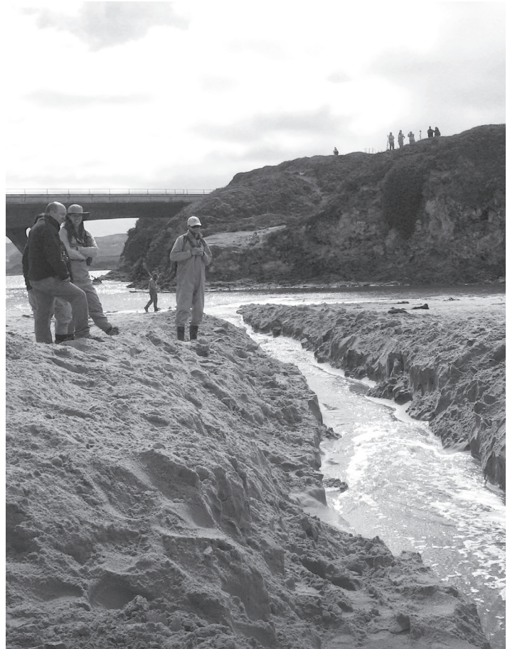
The first attempt: a channel is dug manually
